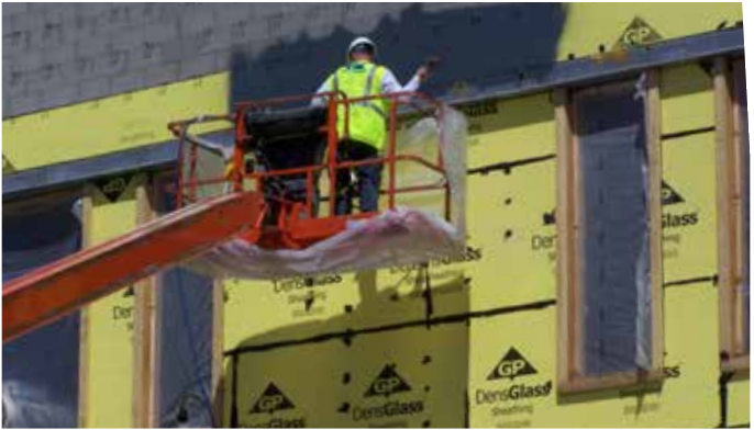
Seams detailed with SUPER SEAL PE™ Joint Sealant
