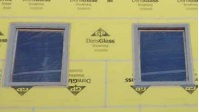
Seams detailed with CLIMATE FLASH™ Flashing Tape
